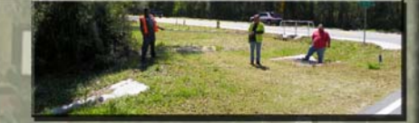
POTENTIAL CONFLICTS WITH DRAINAGE STRUCTURES. AERIAL PHOTOGRAPH BELOW DOES NOT INDICATE RECENT IMPROVEMENTS.
